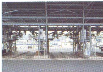
Tanker trucks load and weigh simultaneously on the eight-scale installation at Powell Duffryn Terminals
